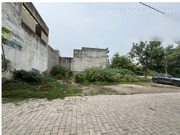
Photo 3. School-side edge of the plot. No independent boundary wall on this side. 14:17.
