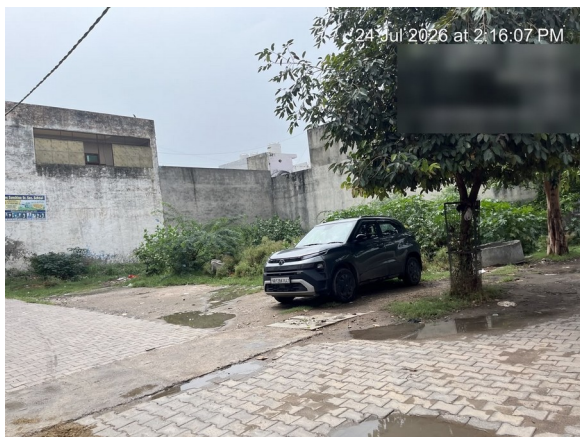
Photo 1. Full plot frontage viewed from the access road; adjoining school building on the left. 14:16.
