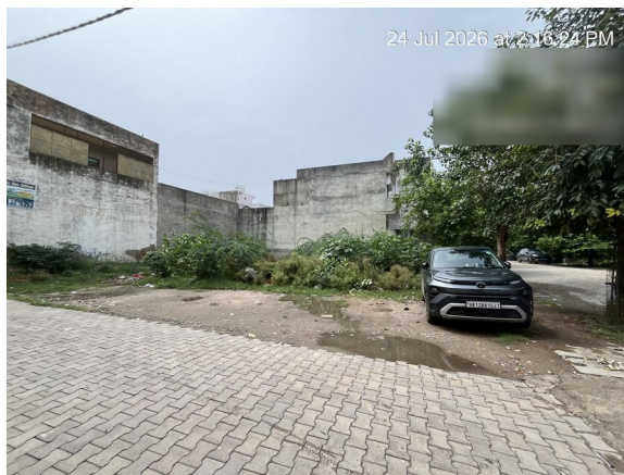
Photo 2. Plot and paved approach from the opposite corner, facing the rear boundary. 14:16.
