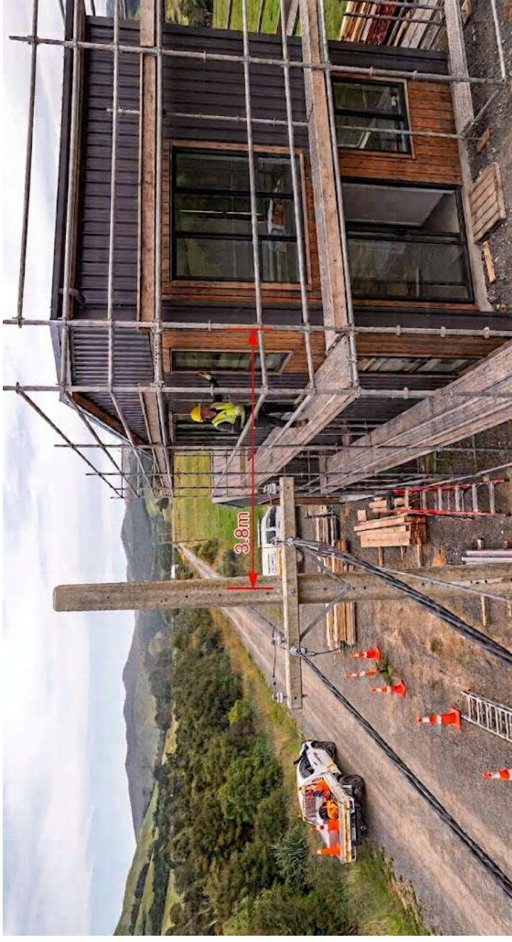
Non-competent scaffold worker able to get within 4m of a cable reticulating on the back of the pole. Engineering assessment required. (AI generated)
