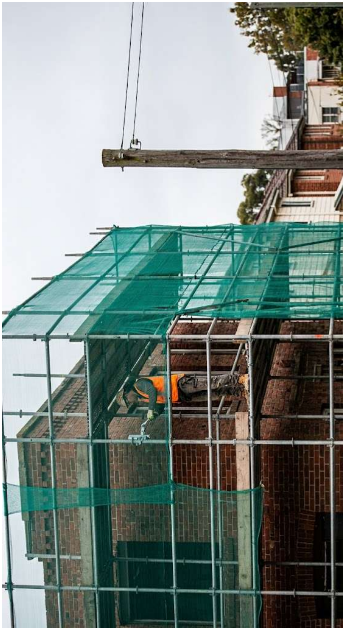
Netting installed to prevent workers being able to access within 4m of the nearest conductor
