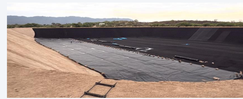
Lining advancing across the basin floor and slopes
