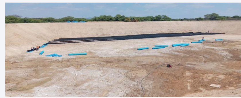
Geomembrane installation — 20 August 2026
