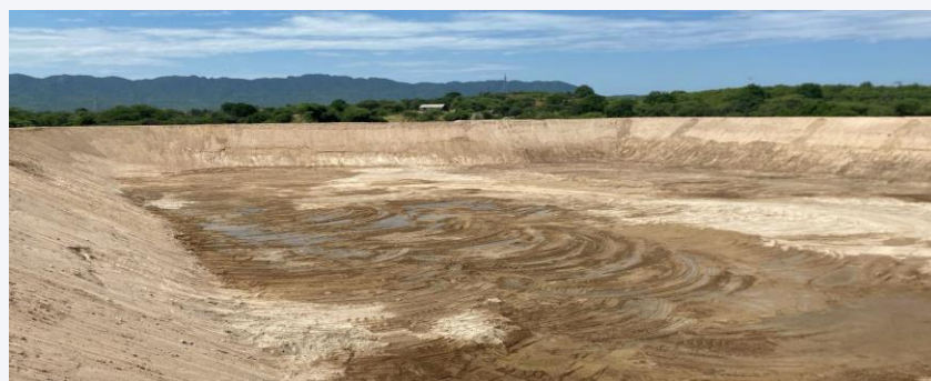
Excavation complete — 10 August 2026
