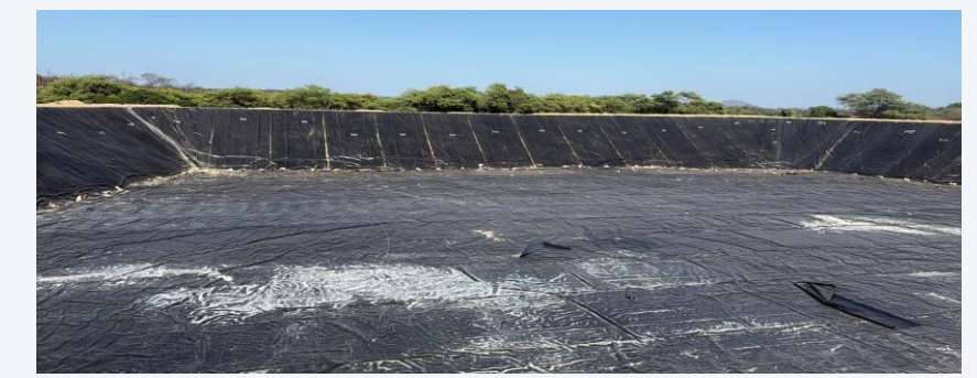
Geomembrane complete — Pond No. 4 inaugurated
