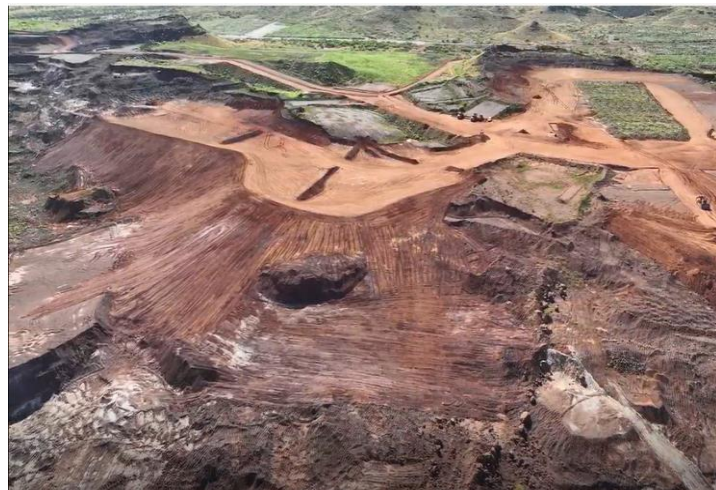
455m RL BATTER AFTER PROFILE LOOKING EAST
