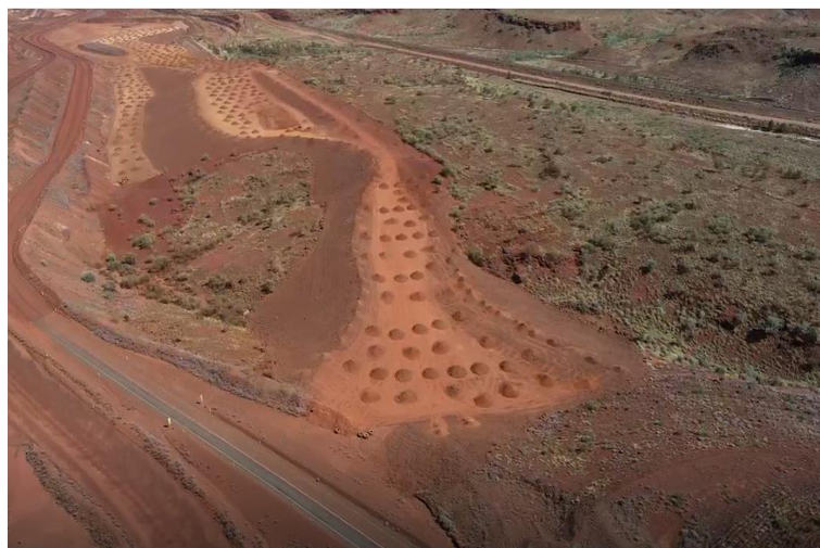
SITE D - BATTER PROFILED/READY TO SPREAD TOP SOIL
