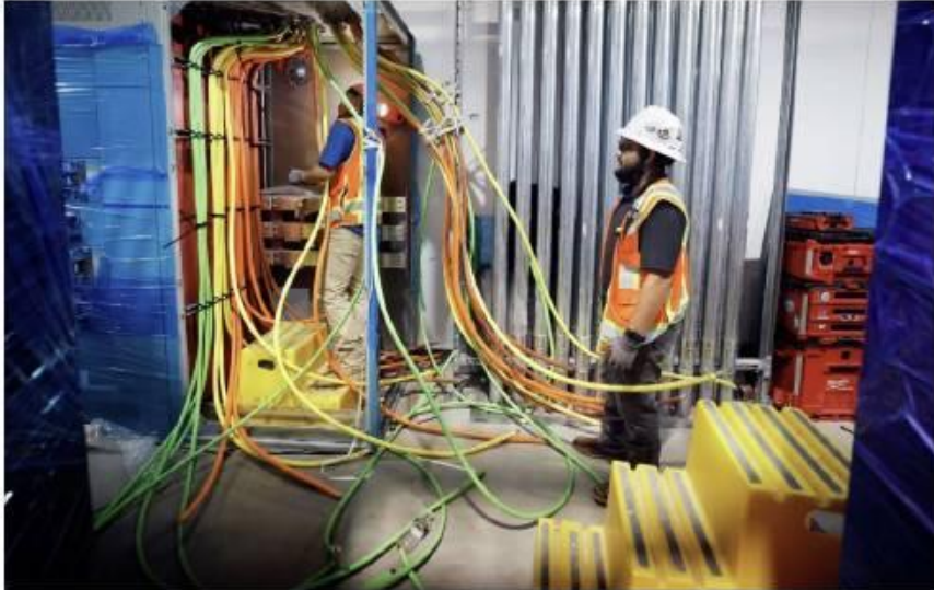
Construction workers wire electricity lines in Dallas TX4 data center's mechanical galley under construction in Garland .
