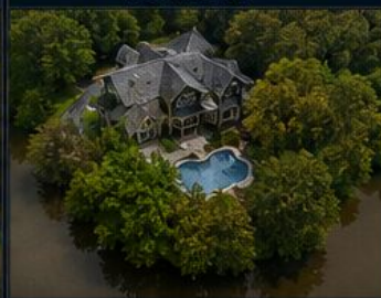
AERIAL VIEW FROM NORTH
