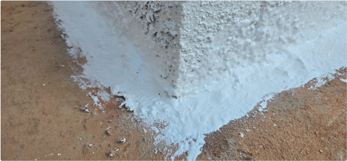
Fig. 1 — Interior wall-to-footing joint sealed with a cementitious waterproof coating before framing begins, carried up the wall and out across the footing so no seam is exposed. Why it matters: this joint is where most basement leaks start — sealing it while the walls are open is the single highest-value waterproofing step in the entire build.
