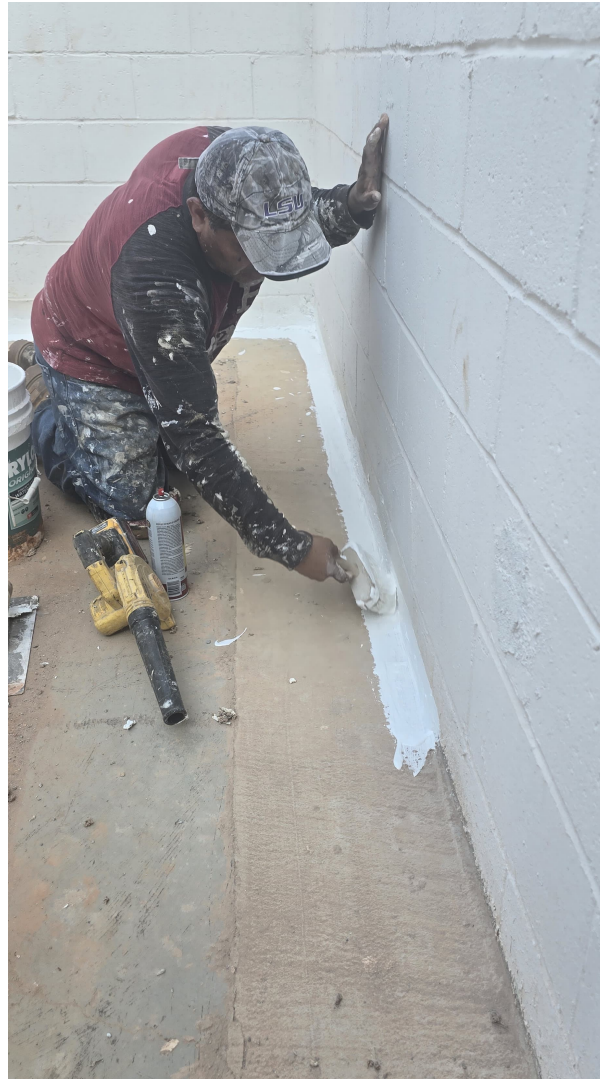
Fig. 2 — A Ducere crew member brushing the cementitious cove coating up from the slab, applying it in the same continuous pass described above so the wall and floor surfaces lap without a gap. Why it matters: hand-brushing the cove, rather than rolling it on flat, is what actually gets full coverage into the corner where the wall meets the floor — the exact spot Fig. 1 shows finished.
