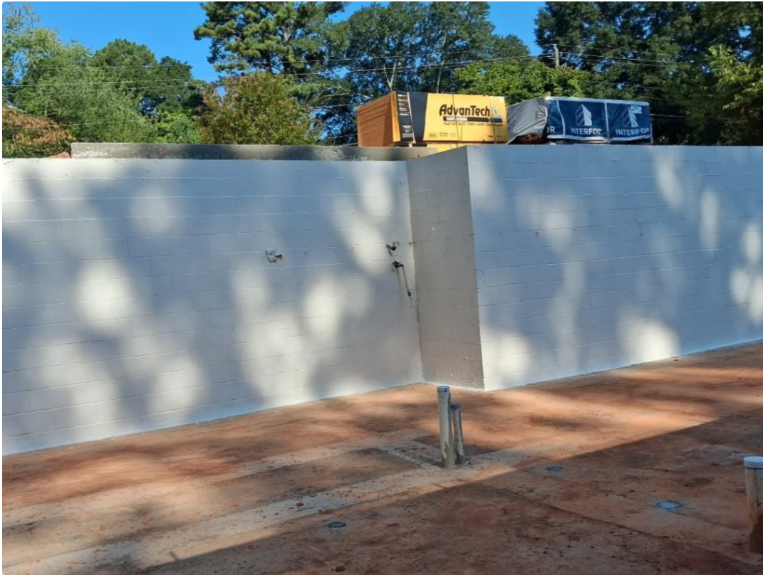
Fig. 3 — Exterior CMU foundation wall fully coated with a waterproof membrane, photographed before backfill and framing. Why it matters: once soil goes against this wall, the coating is on duty with zero margin for missed spots — Ducere applies it while every square foot is exposed and inspectable.
