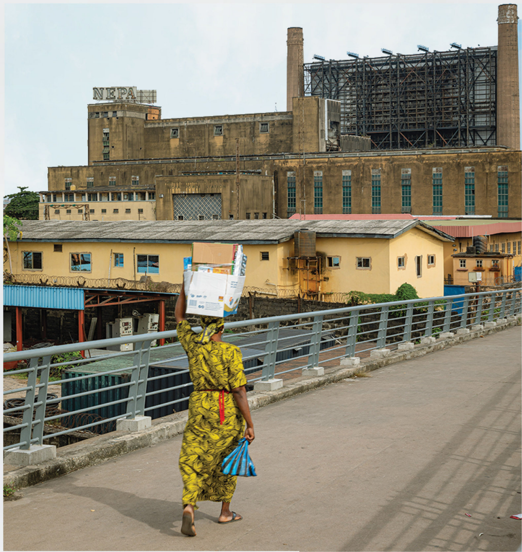
Ijora Power Station - Existing View
