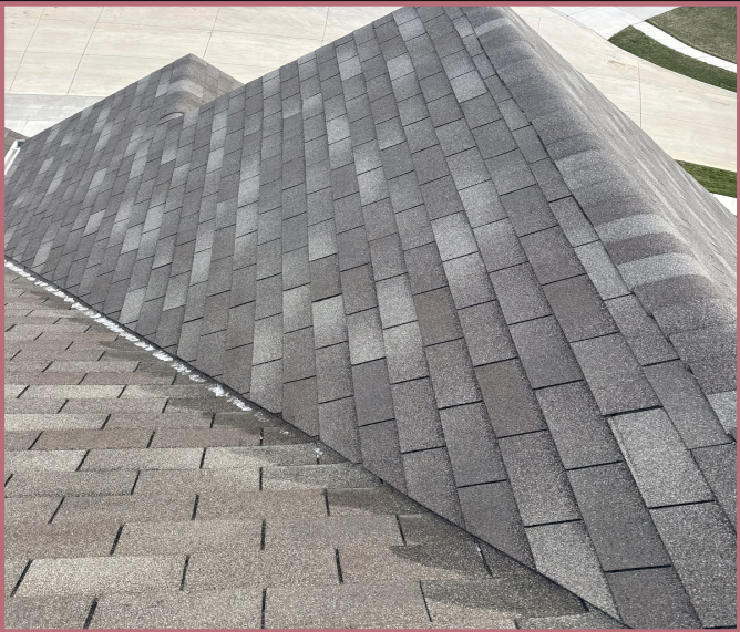
House - Right Slope - Overview
