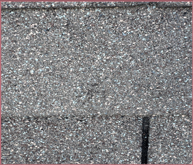
House - Front Slope - Roof Condition
