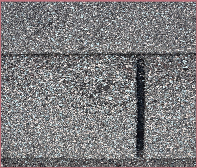
House - Right Slope - Roof Condition
