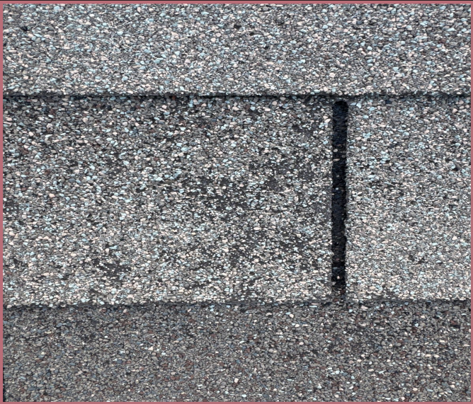
House - Back Slope - Roof Condition
