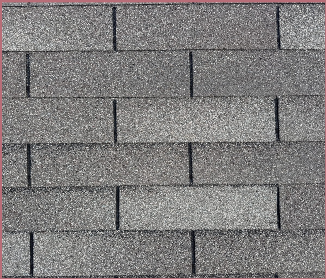
House - Left Slope - Roof Condition
