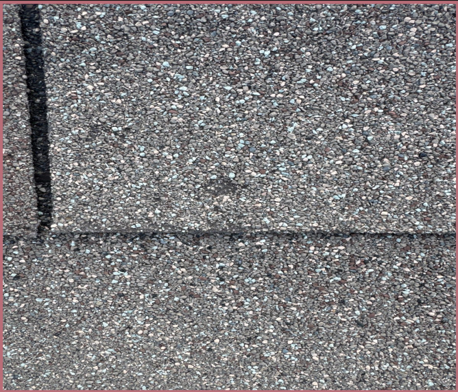
House - Back Slope - Roof Condition
