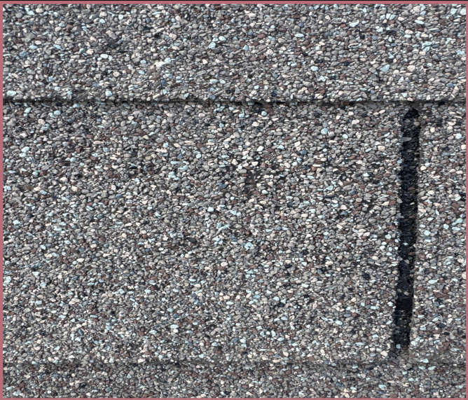
House - Right Slope - Roof Condition
