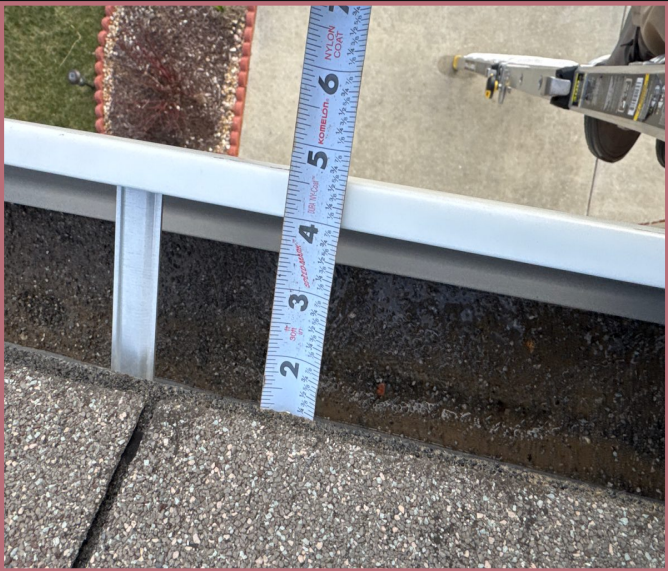
House - Gutter size measurement
