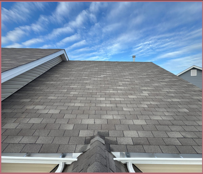
House - Front Slope - Overview
