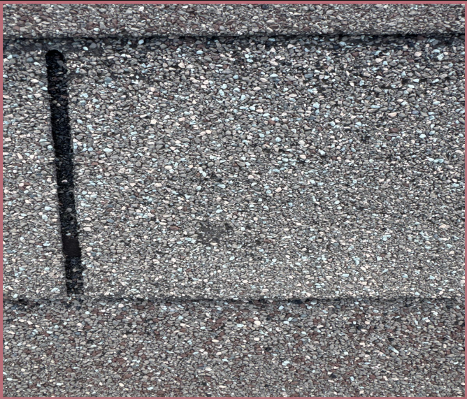
House - Back Slope - Roof Condition
