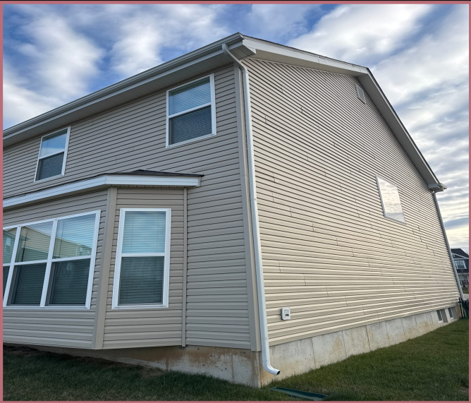
House - Back Elevation - right corner measurement
