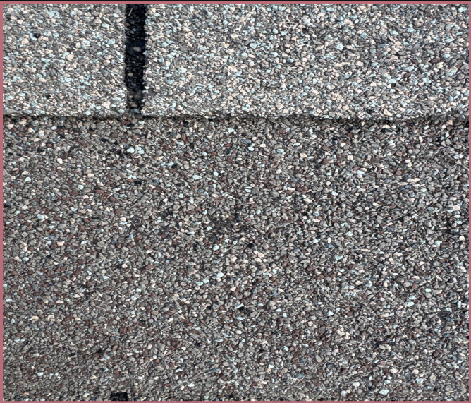
House - Left Slope - Roof Condition
