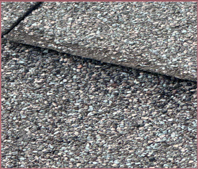
House - Right Slope - Roof Condition
