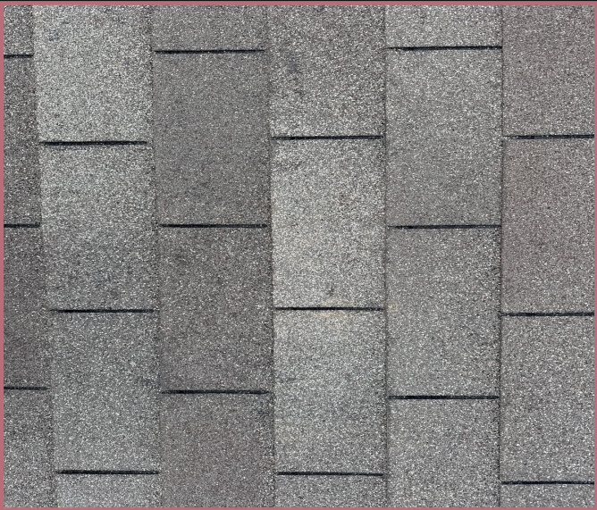
House - Front Slope - Roof Condition
