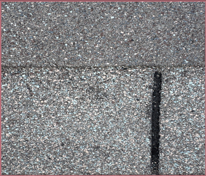
House - Front Slope - Roof Condition
