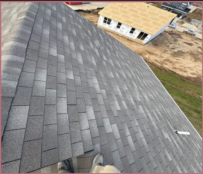
House - Back Slope - Overview
