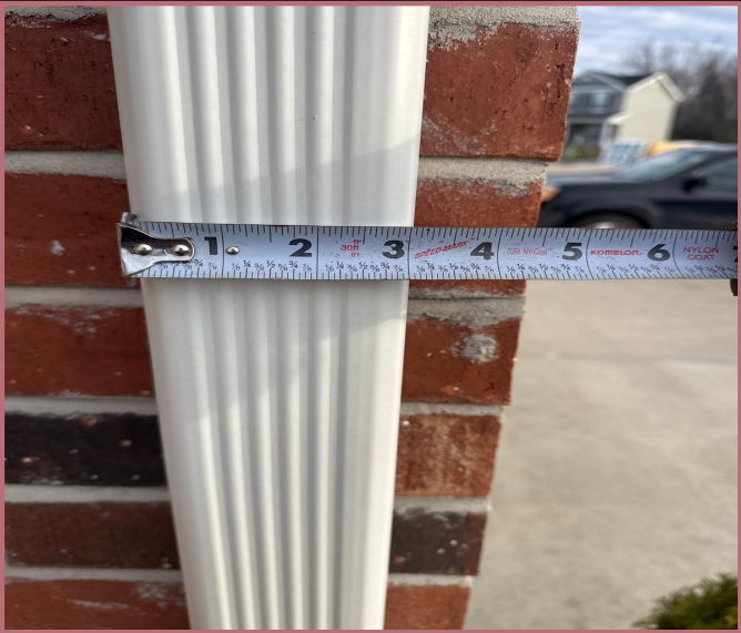
House - Gutter size measurement
