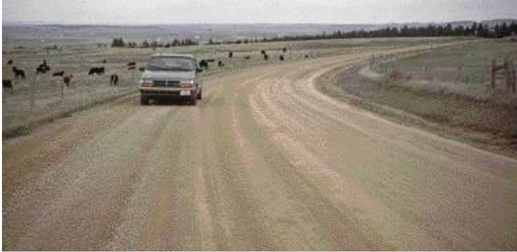
This superelevated road section makes driving safer.
