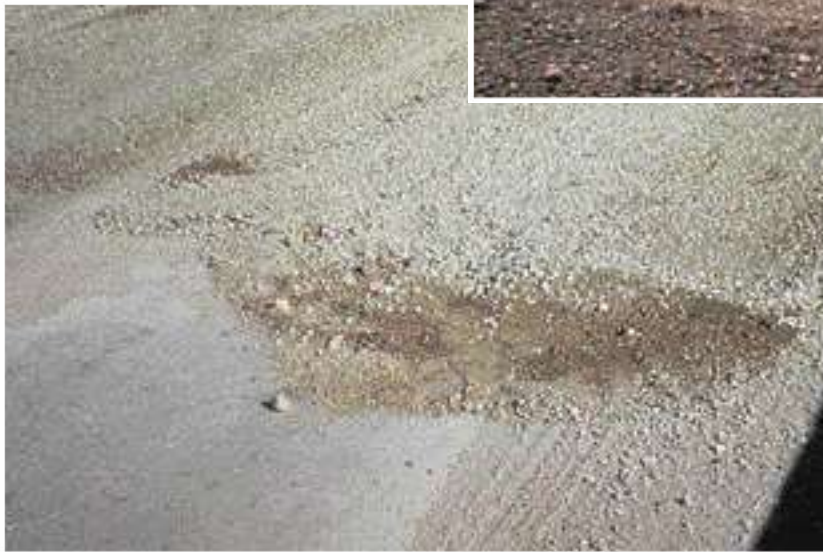
Nice job of blade work to shape road to match bridge deck.
