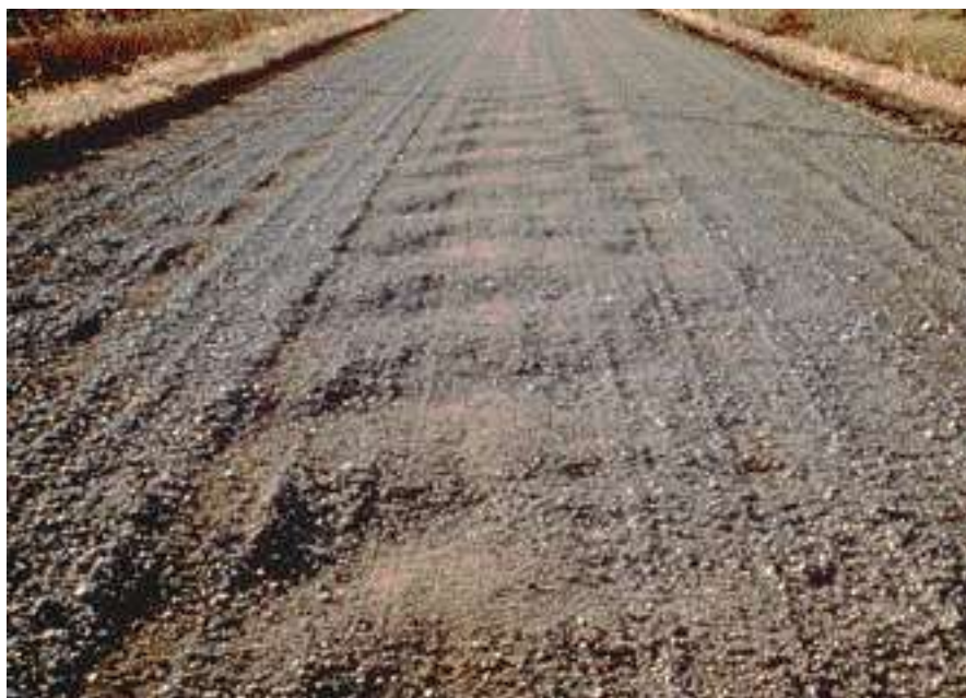
This type of washboarding appears at an angle across the roadway with ridges and depressions two to three feet apart. It is caused by excess grader speed.
