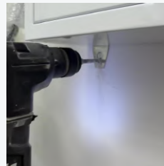
DRILL LOWER HOLES
