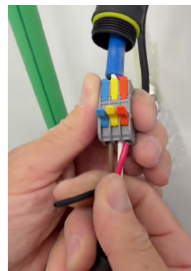
MATCH + INSERT WIRES
